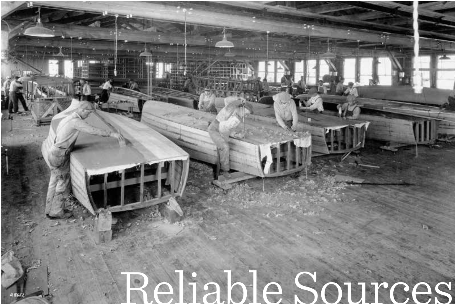
Factory production of mahogany boats at the company that would become Chris-Craft, in Algonac, Michigan, in the early 20th Century. Photo courtesy of Chris-Craft
